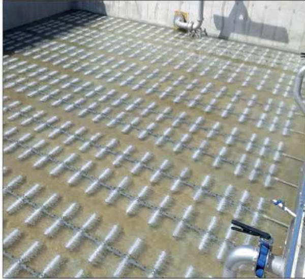
AirRex® piping system with MAGNUM® tube diffusers
